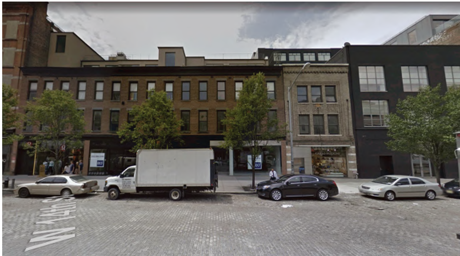
VIEW FROM 14TH STREET, NORTH SIDE OF STREET
