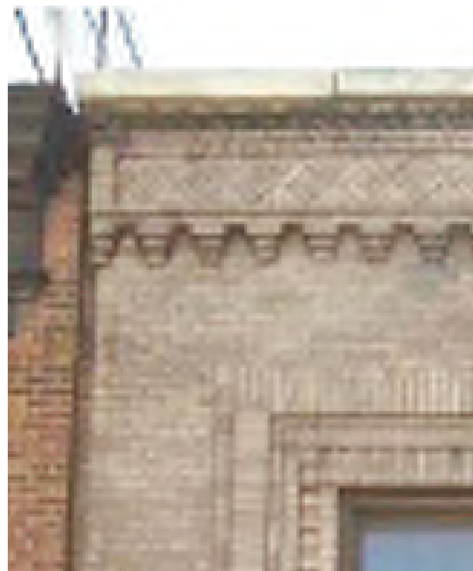
FRAME AND MARBLE CORNICE DETAIL
