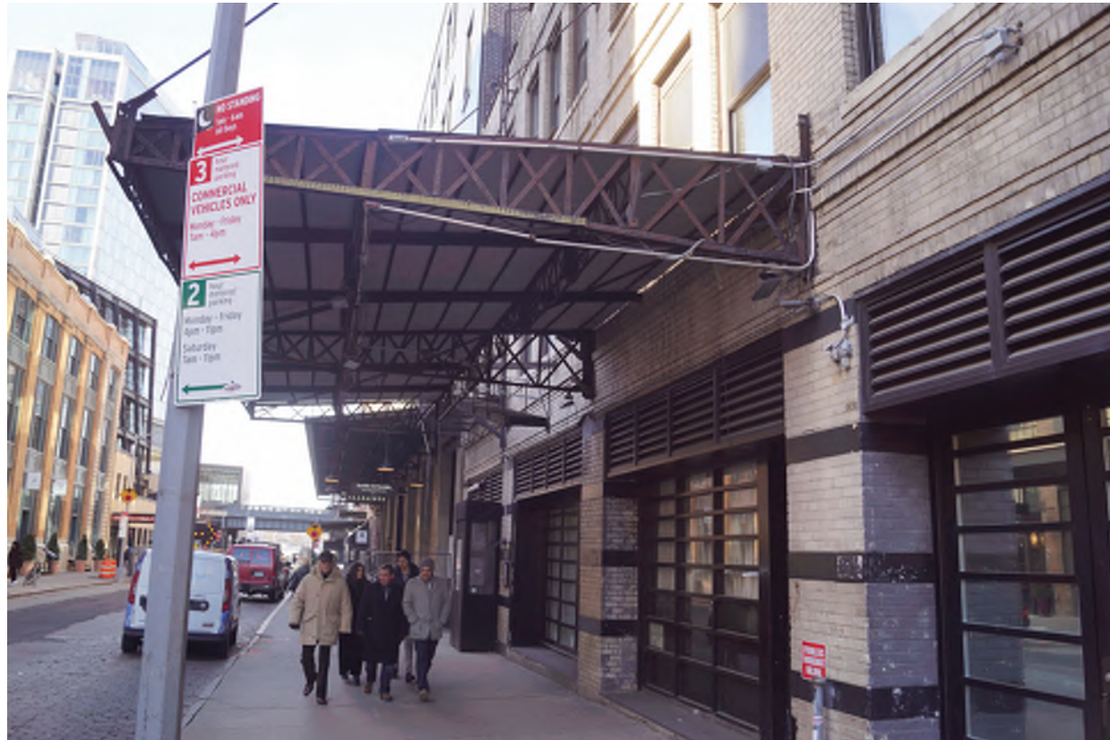
EXISTING STOREFRONT AND CANOPY
